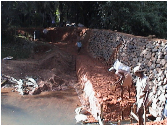
Fig. 3 – Construction of temporary check-dam underway.
