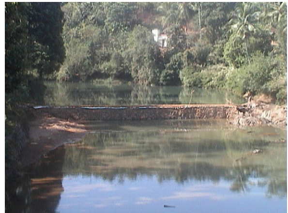
Fig. 1 – Temporary check-dam built across a seasonal stream in the Kumbadaje panchayat.
