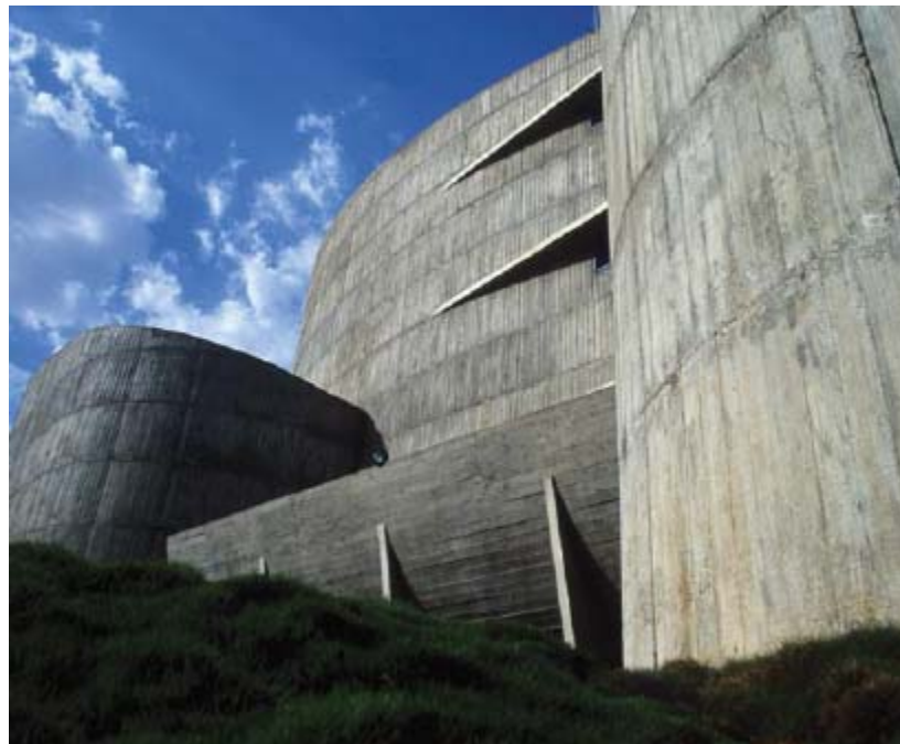
Figure 2. The slightly hermetic concrete exterior of Prathama
